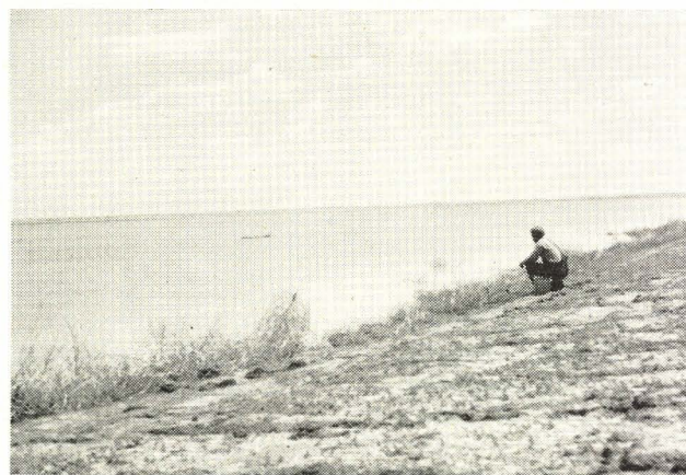
May rains brought water pouring into Cheyenne Bottoms, waterfowl refuge in Barton county. The top picture shows the inlet canal running bankful. Below the water from the Wet Walnut creek boils through a drop structure into the inlet canal. Third picture, a fisherman tries his luck in the rain-enlarged main pool.
